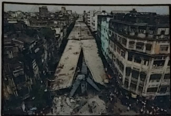
Pic.- Vivekananda Road Flyover
